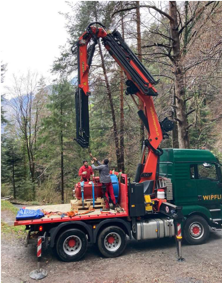
Transport Turbine zur Revision
